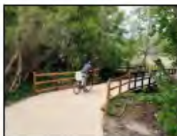
An aggregated shared footway/cycleway exiting development onto Cockham Lane
