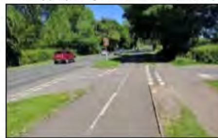
Shared footway/cycleway connecting to Ockham Park roundabout from west of development
