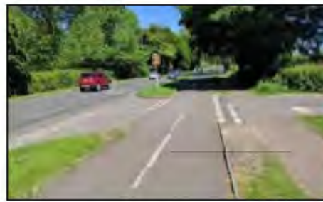
3m Shared footway / cycleway along Wisley Lane diversion and across Ockham Park Roundabout
